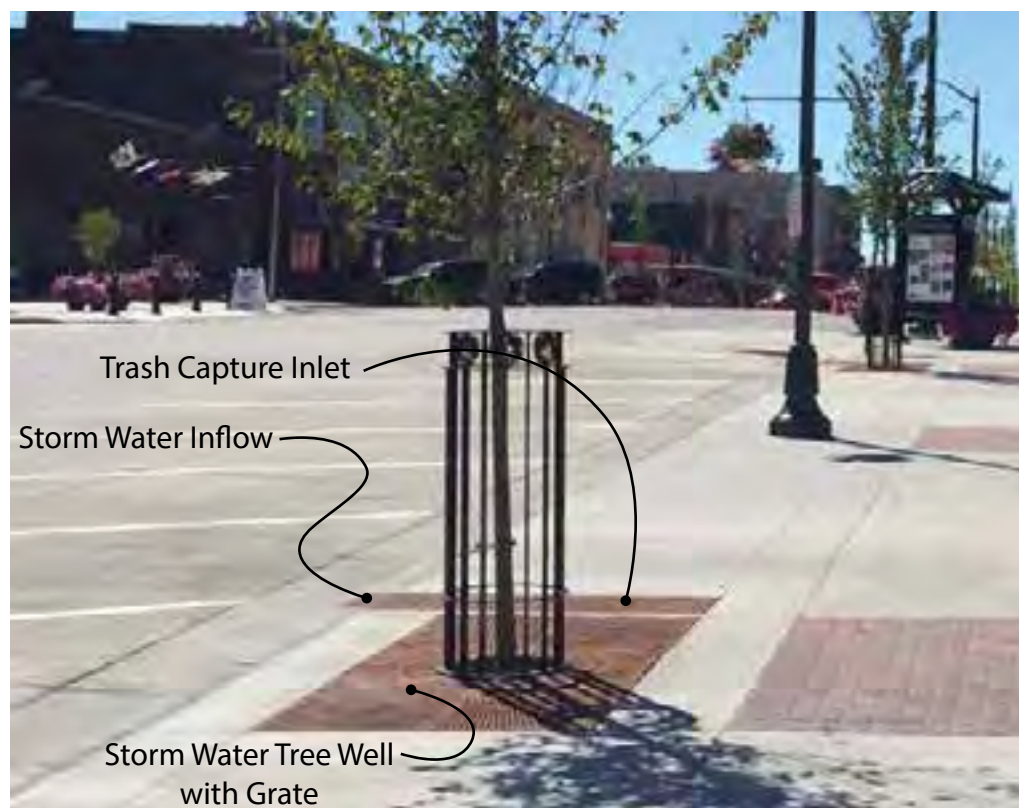
TYPICAL SECTION: STORMWATER TREE GRATE THROUGH TREE SCALE: 3/8" = 1'-0"
