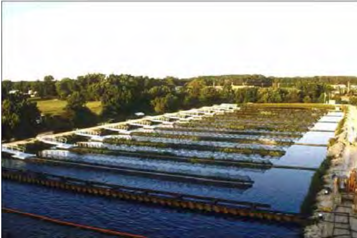
Tyson Restorer-based treatment system, Berlin, Maryland
