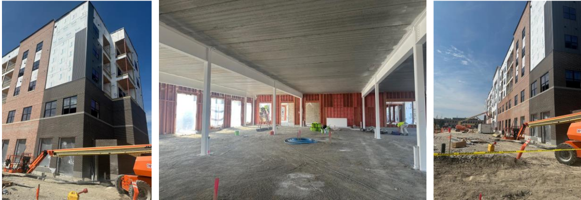
Figure 2. Park – Stage Concrete & 151 Lofts (Background)
