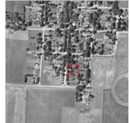
1950s Historic Aerial Photo
