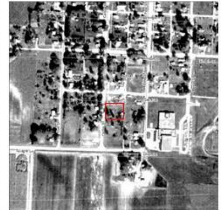
1970s Historic Aerial Photo
