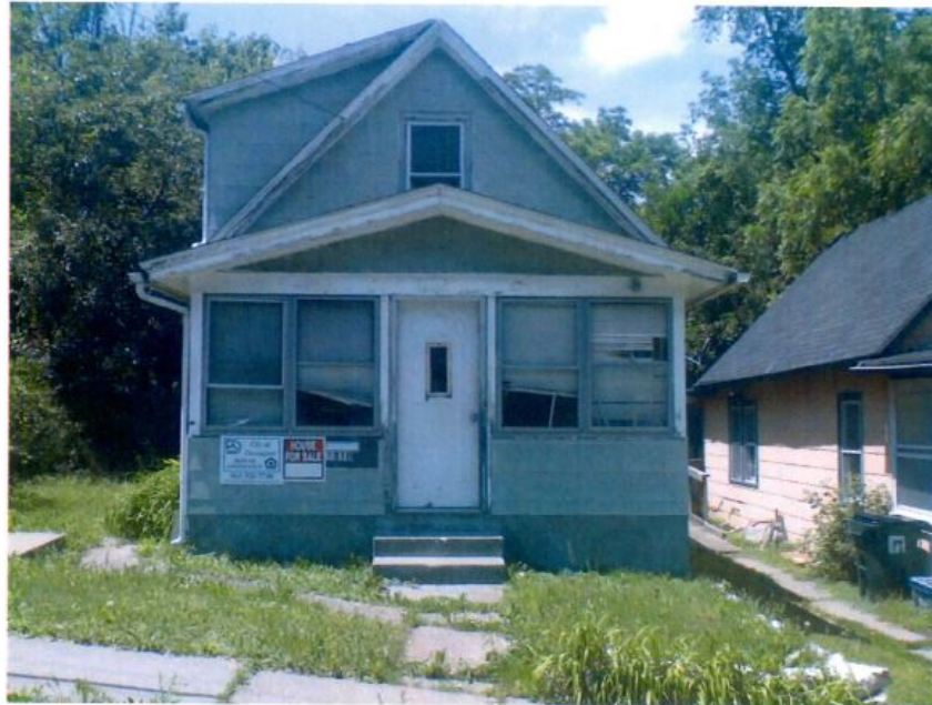
Front of 1310 Eastern, facing west
