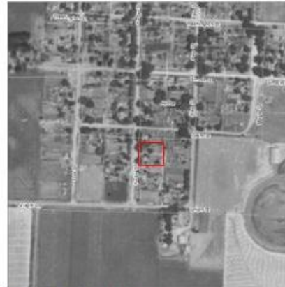
1930s Historic Aerial Photo
