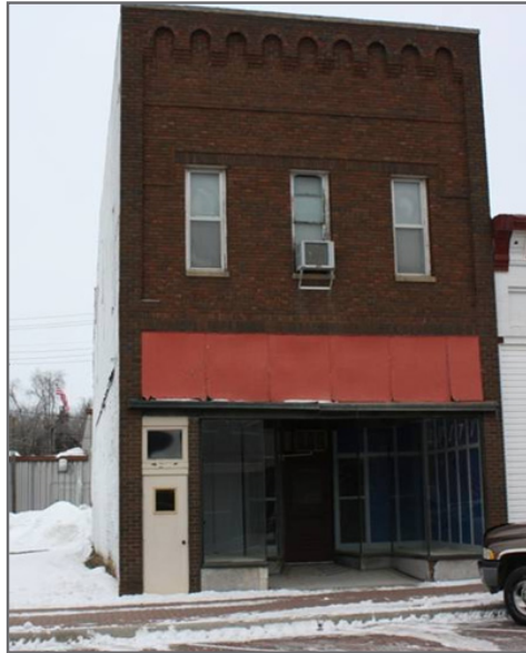
Fig.4 Pre-Retrofit Energy Usage: 96,600 BTU / Sq Ft / Yr Post-Retrofit Energy Usage: 67,200 BTU / Sq Ft / Yr
