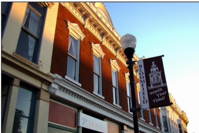
Upper story housing is part of the rehabilitation efforts in Bloomfield
