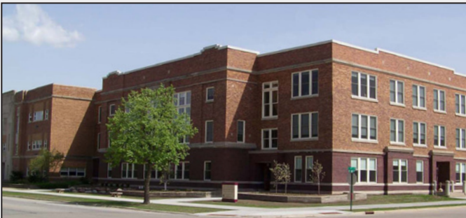
Spencer historic school building with 16 units of affordable housing
