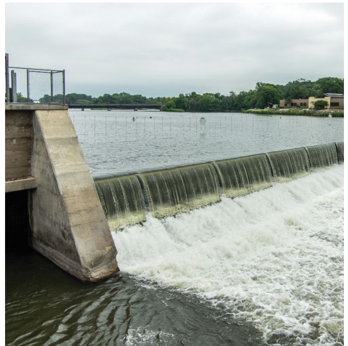
Waverly's inflatable dam, completed in 2011, automatically adjusts its height to maintain a set water elevation.
