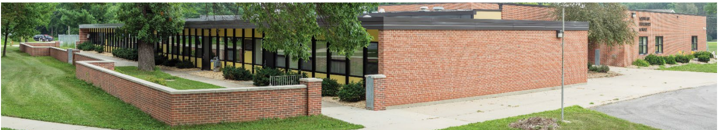
Waverly's Southeast Elementary School is now protected by a 4.5 foot flood wall.
