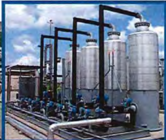
Biomethane System Equipment. Located inside the current engine room for cold weather protection and ease-of-maintenance.
