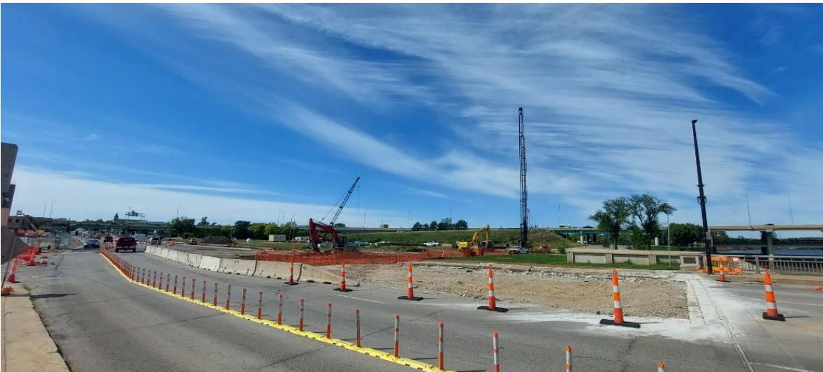
1 st Avenue SW – Public Right of Way Improvements
