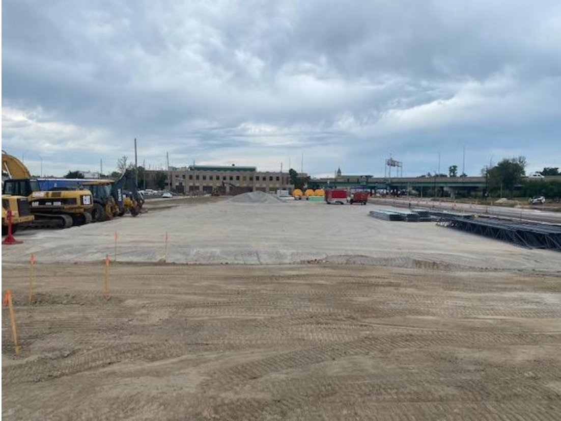
Utility Work - Mass Grading – Phases 1 and 2
