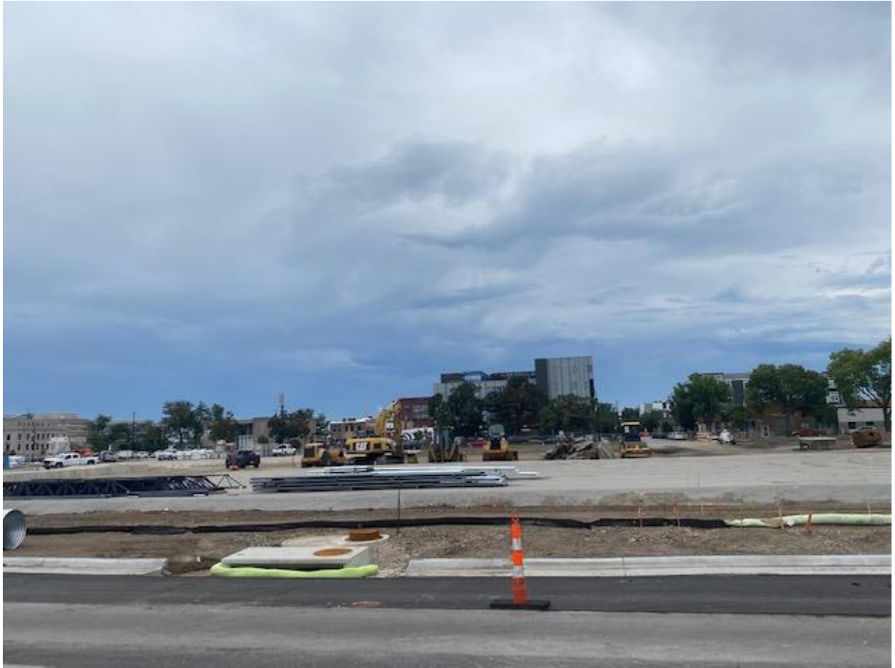
Mixed Use Building Pad - Materials Stored for Pickle Palace – Phase 1
